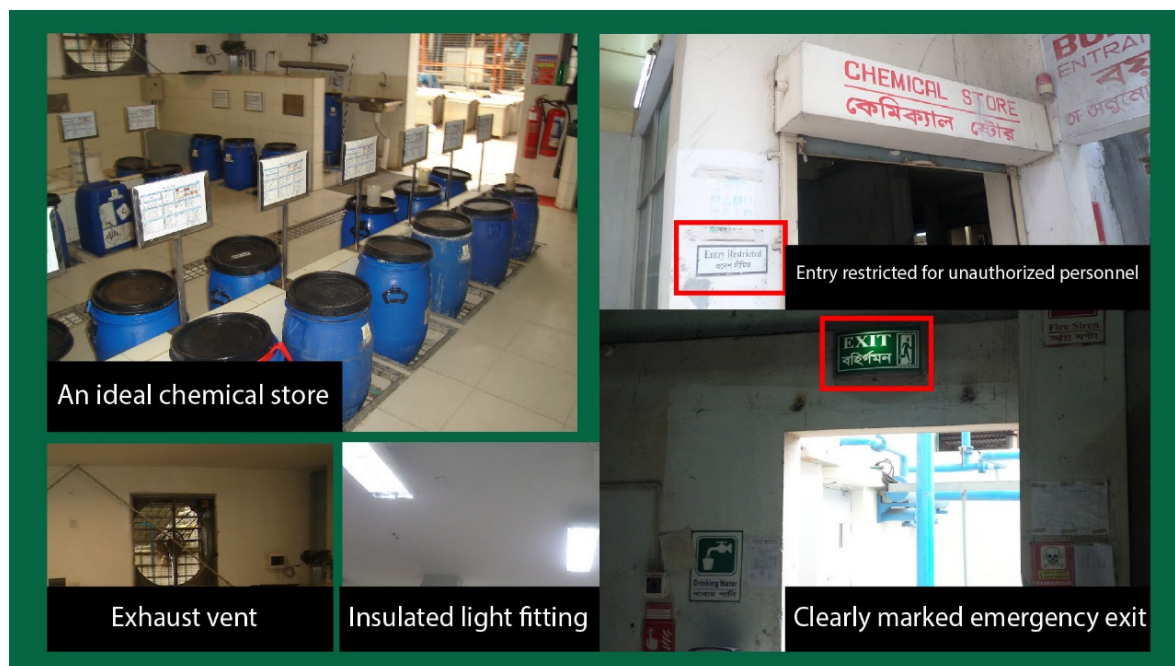
Figure 3: Safe chemical storage - Structure, layout and size of chemical store. Photo source: Reed Consultancy Bangladesh. Collaged courtesy: Kazi Farhan Hossain Purba.
